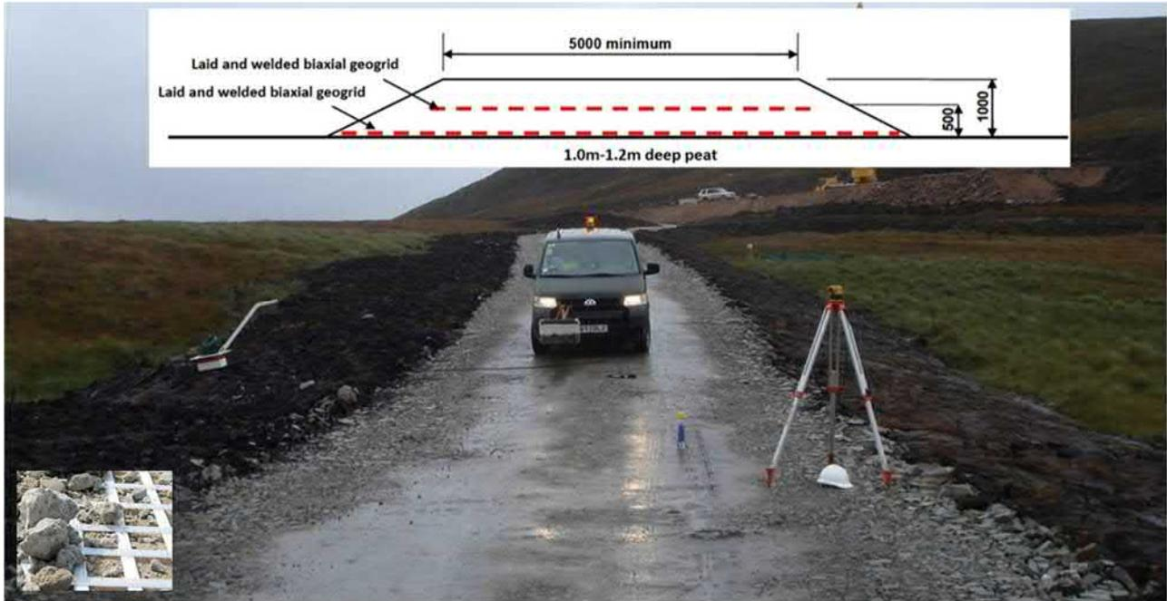
**Figure 1: Designed and constructed geogrid reinforced floating road on a peat in a Scottish windfarm (SNH, 2010)**
