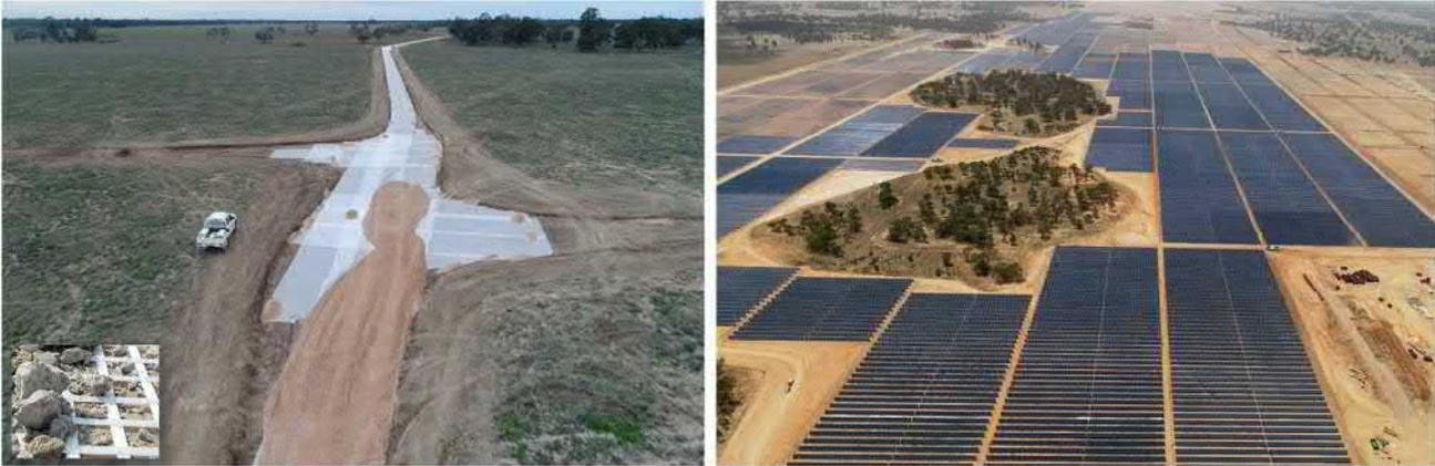
**Figure 22: Darlington Point solar farm, Australia-geogrid reinforced access roads during construction (a-left) and after completion (b-right, <https://edifyenergy.com/project/darlington-point>)**
