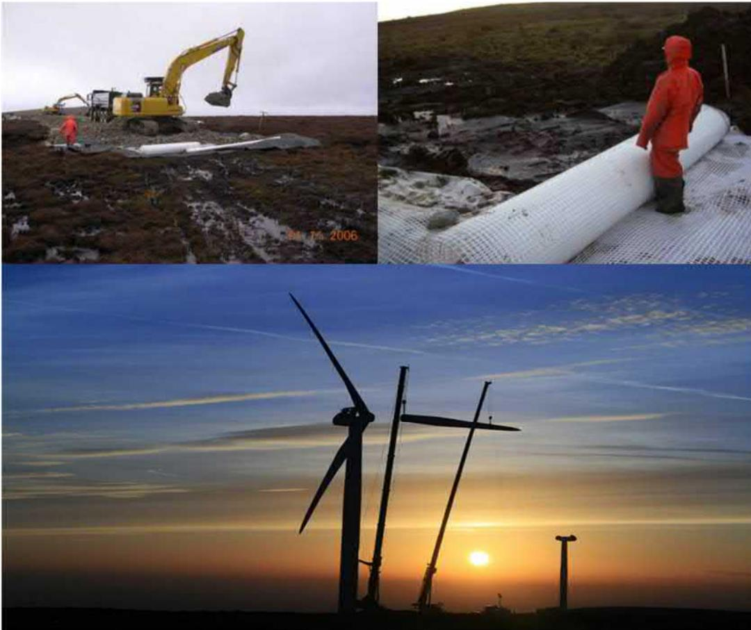
**Figure 17: Scout Moor windfarm, UK- construction of geogrid reinforced access roads and hardstands (top) and installation of the wind turbines (bottom, <http://www.peelenergy.co.uk>)**
