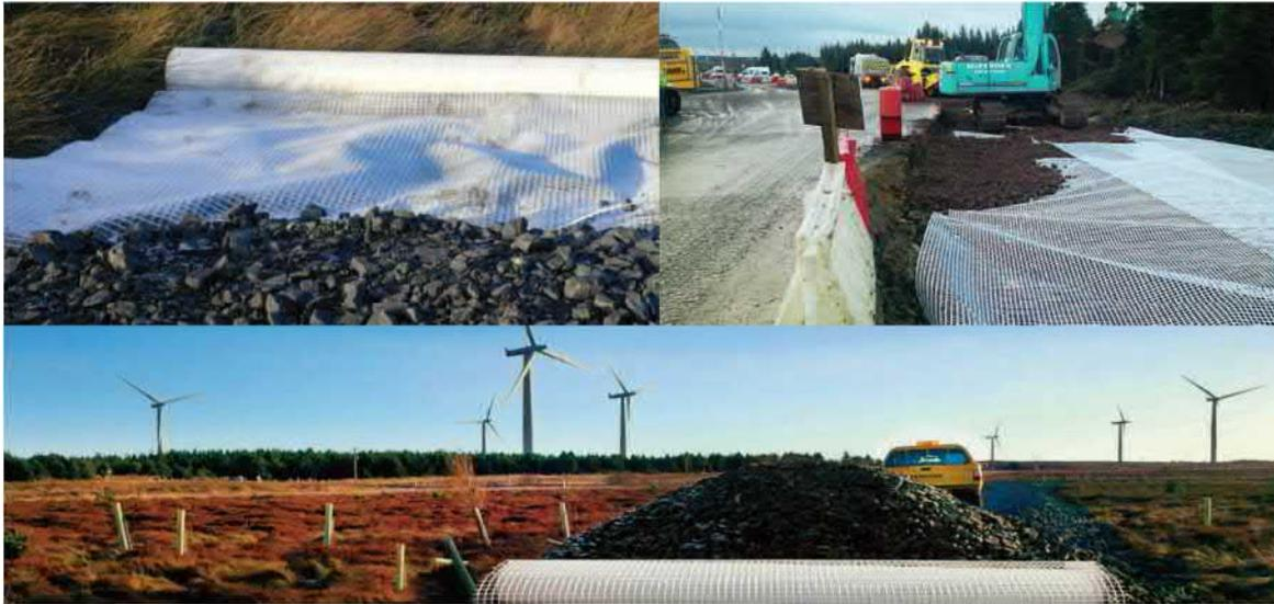
**Figure 18: Black Law windfarm geogrid reinforced access roads and hardstands construction-Combigrid laid and welded biaxial geogrid-geotextile composite on the subgrade (top left) and laid and welded biaxial geogrid intermediate reinforcement (top right and bottom)**
