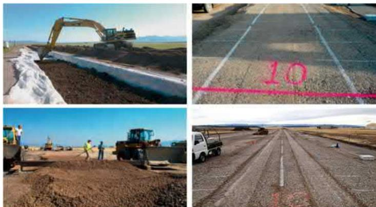
**Figure 5: Geogrid reinforced unsealed road full-scale field trial: from construction stage to end of trial (Cuelho et al., 2014)**
