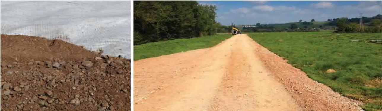
**Figure 20: Redlands solar farm Combigrid geogrid-geotextile composite reinforced access roads**
