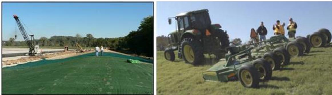
**Figure 4 Left: Installation of the HPTRMs on the levee (Sphat, 2012b), Right: Maintenance equipment used in the field trial (Thompson and Loizeaux, 2018)**
