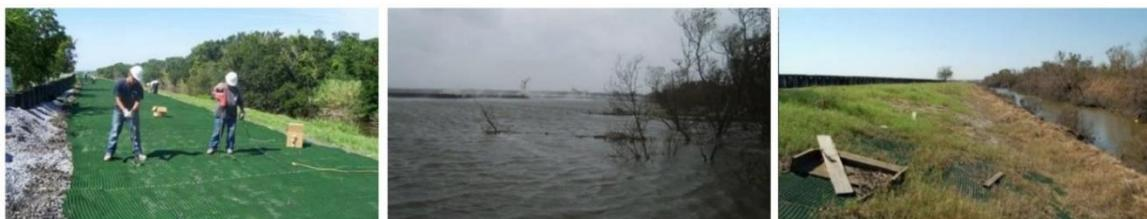
**Figure 3 Armormax® EEAS on Penn Levee (left), Stormwater overtopping Armormax® armoured Penn levee (middle), Successful performance of Armormax® EEAS after the storm (right) (Thompson and Loizeaux, 2018)**
