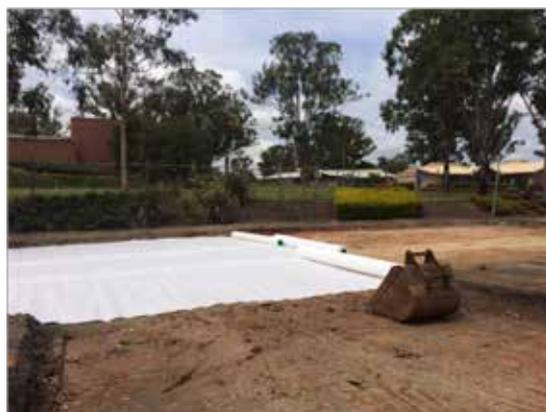
Photo 2 - Use of Combigrid 30/30Q1 to provide reinforcement and separation in one product!
