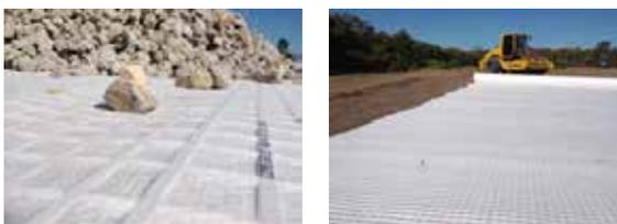
Through using the high stiffness reinforcement and separation benefits of Combigrid® and the reinforcement of Secugrid®, the client achieved a considerable time and cost saving, using less granular material and a more efficient geosynthetic product than originally specified.
