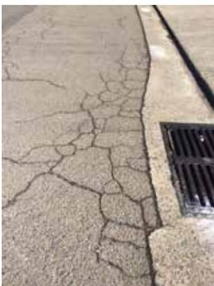
Photo 1 - Typical flexible asphalt pavement “crocodile cracking”
