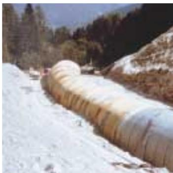
Secudrän® in a tunnel application (Pustertal, Italy). Precipitation and groundwater are drained
