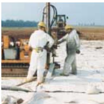
Installation of Secudrän® prefabricated vertical drains to accelerate consolidation
