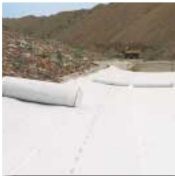
In landfill applications, Secudrän® completely drains leachate or precipitation
