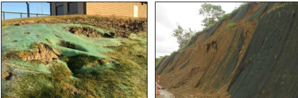
**Figure 7 Surficial Slope Instability**
