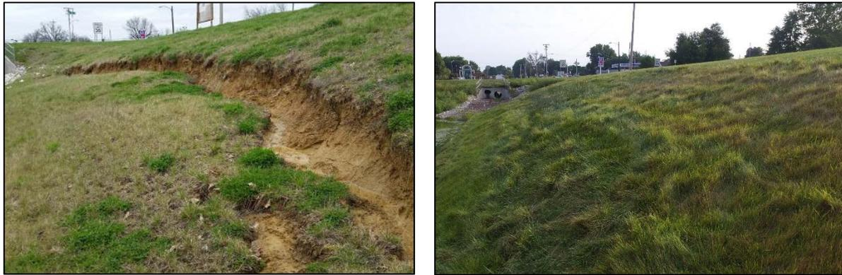
**Figure 9 Surficial Slope Failure (Left) stabilized with EEAS (Right)**
