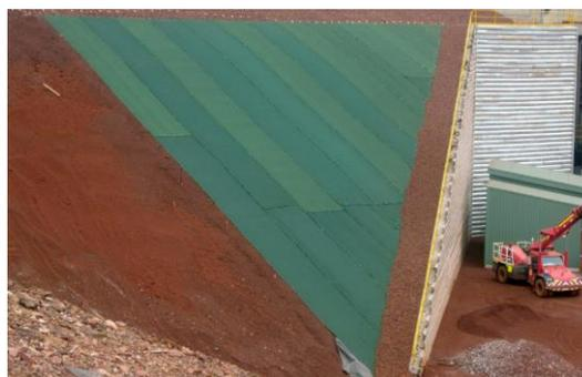
**Figure 4. Installed TRM3 on the slope, King Solomon, WA**
