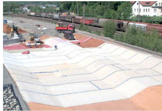
Figure 2 Bentofix® X sealed section and cover soil placement
