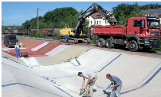
Figure 1 Taping of Bentofix® overlaps
