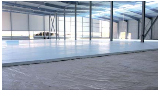
Figure 3 Insulation placed directly over the coating side of Bentofix® X
