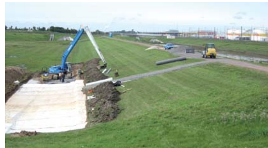
Figure 6 Cover soil placement over installed Bentofix® GCL
