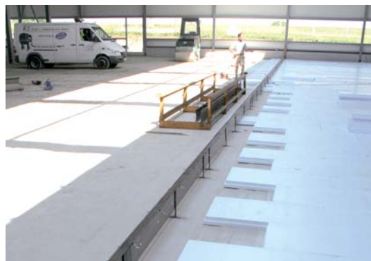
Figure 4 Preparation for the concrete pouring over Bentofix® and insulation
