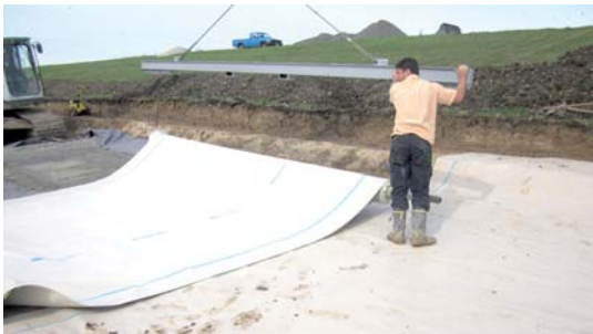
Figure 5 Installation and overlapping of Bentofix® X GCL rolls
