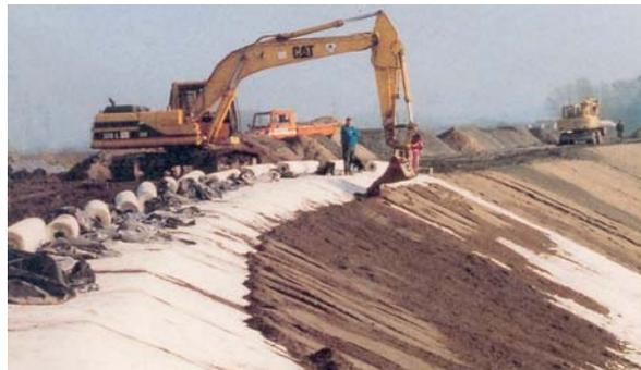
Fig. 4 Lippe River levee reconstruction (1994): Installing Bentofix® GCL as a levee seal (Saathoff & Werth 2003)
