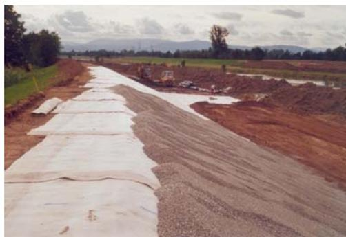
Fig. 3 Covering Bentofix® GCL with locally available fine gravel to ward off burrowing animals
