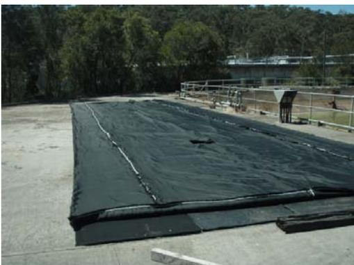
Photo 8 Positioning the geotextile tube.
