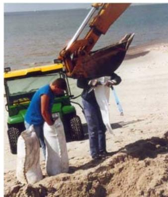
Photo 7 Filling Geotextile Bag
