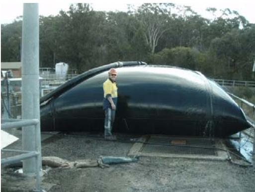
Photo 10 Geotextile tube filled
