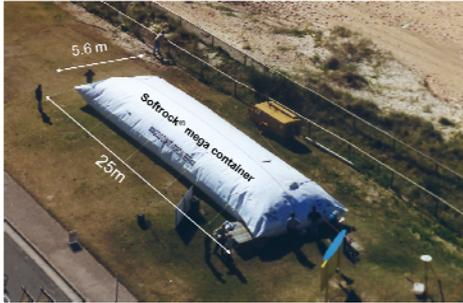
Photo 4 Geotextile Container
