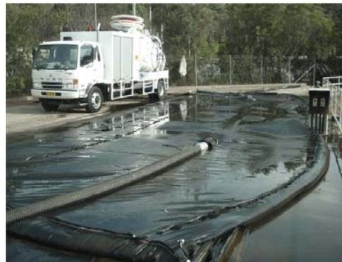
Photo 9 Filling of geotextile tube commences
