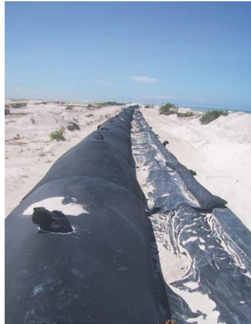
Photo 3 Geotextile with Scour Apron
