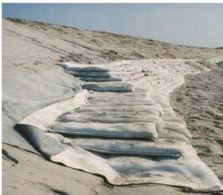
Photo 6 Geotextile Bag Placement.
