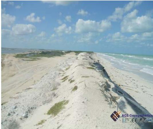
Photo 1 Geotextile Back Beach Protection.
