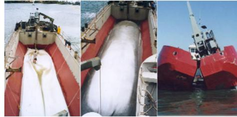
Photo 5 Geotextile Container in Barge
