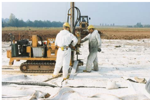
Figure 7 Installation of vertical drains
