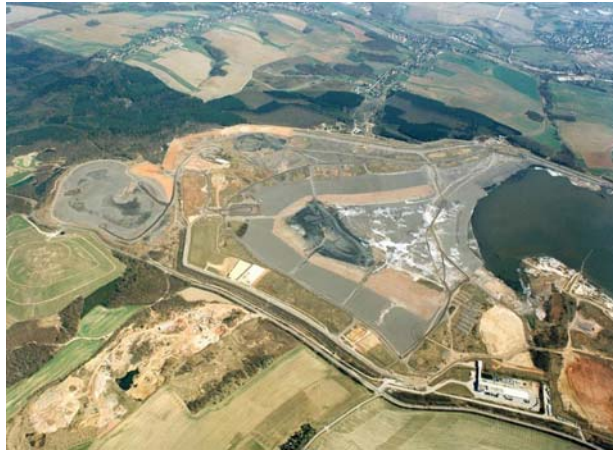
Figure 6 Aerial view of a Tailings Management facility
