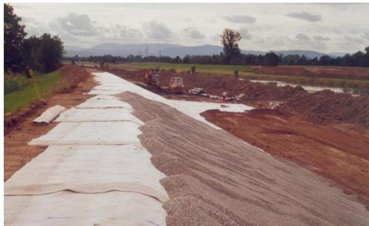
Figure 8: Rehabilitation of the Kinzig river levee in 2001 with GCL - installation of non-cohesive river gravel as cover soil for the GCL (Heerten et al., 2008)
