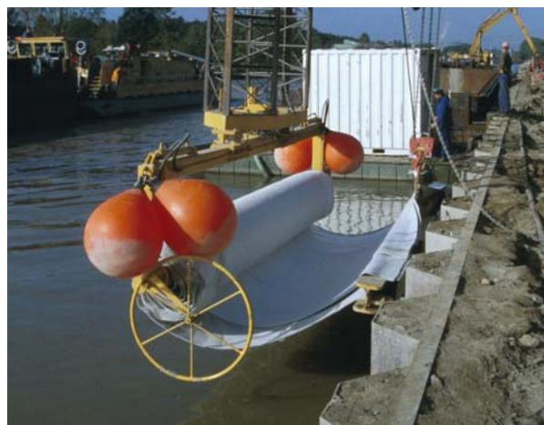
Figure 4: GCL and sand mat separately enrolled on a spreader bar as lining system for underwater installation (Fleischer & Heibaum, 2002)
