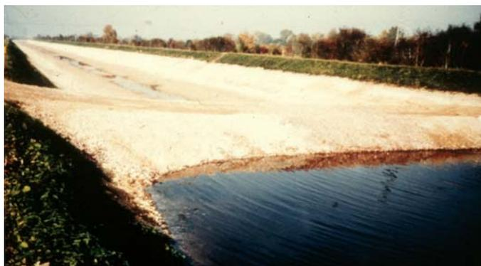
Figure 1: Rehabilitation of the hydropower canal Lech in 1989 – easy coffer dam lining with GCL
