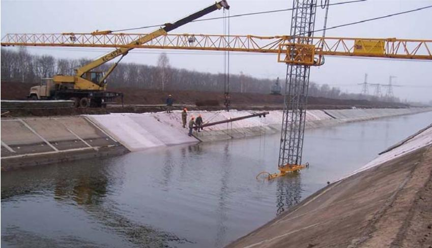
Figure 5: Underwater installation of the sand mat and GCL composite in a drinking water canal in the Ukraine, 2004
