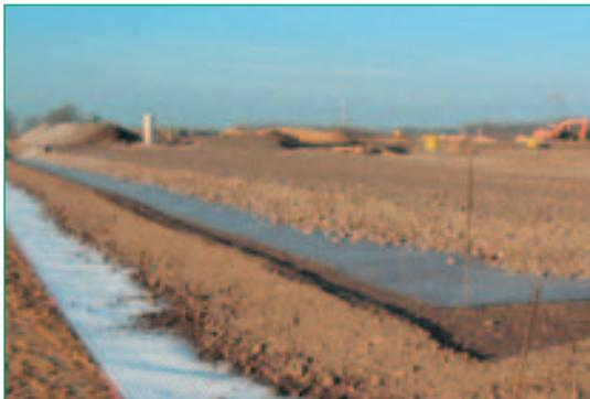
About 7,000 m<sup>2</sup> of Combigrid® 60/60 Q1 251 GRK 4 were used as the bottom reinforcement layer. Combigrid® ensured the separation and filtration between the embankment's bulk material and the finely grained subsoil along with providing the first layer of soil reinforcement.
