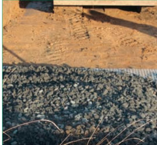
then tested using a plate load test to determine the resulting bearing capacity of the subsoil. Control sections were also built where the thickness of the base course, without geogrid reinforcement, were 300 mm and 400 mm thick. Three different geogrids were incorporated in the study and were installed in the geogrid reinforced base course sections as follows.
