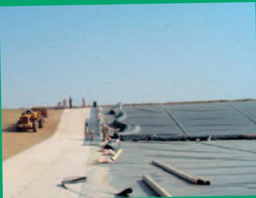
A protective embankment and layer of rockfill was created at one end of the tailing facility to slow down the flow of tailing sand pouring into the tailing pond. A separation layer of Secutex® R304 was specified for this area prior to the positioning of the rockfill and also below the drain material and the drainage pipes. The lining work was carried out by Trading and Development Partnership who are NAUE's approved installer in Saudi Arabia. The work was completed in 13 weeks.
