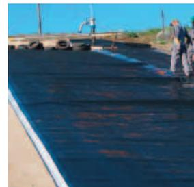
**Fig. 3:** Installed Carbofol® geomembrane with overlap protection strip on a landfill cap (Ämmässuo, Finland)
